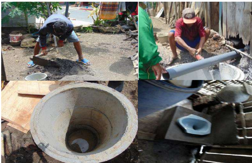
Fig. 4. The process of installing the latrine at Mr Musahid's house
