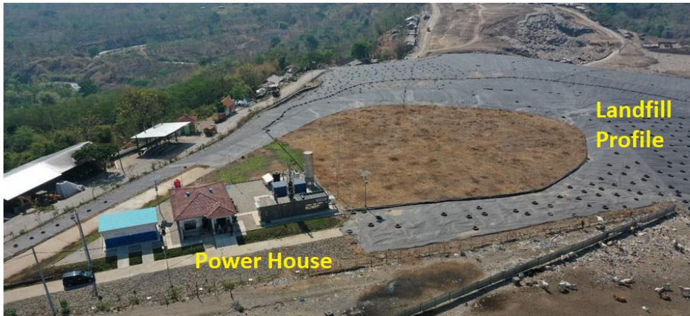
Figure 1. Landfill Gas Power Plant - PLTSa Jatibarang, Semarang
