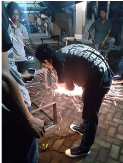
Figure 3. The process of handwashing media construction
