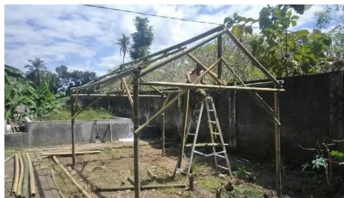
Figure 7. Greenhouse construction process.
