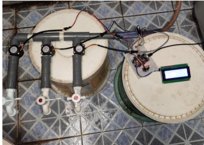
Fig 1. The taps and their water flow sensors
