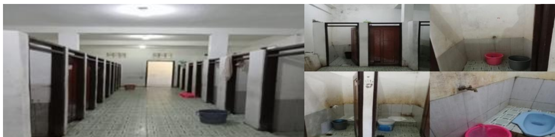
Fig 1. Sanitation facilities at the Islamic boarding school (11 bathrooms and 7 toilets)
