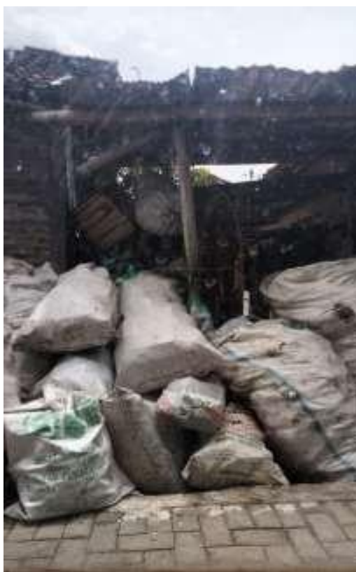
Fig 2. Conditions Around the House
