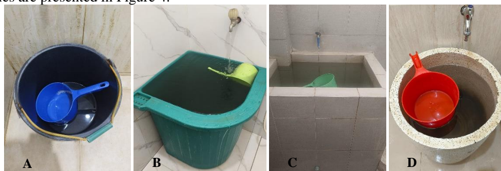
Figure 3. Water storage facilities in the 44 observed mosques. The images are arranged based on the most dominant quantity. A. plastic bucket (n = 17), B. plastic tank (n = 16), concrete tank (n = 10), and concrete pot (n = 1).
